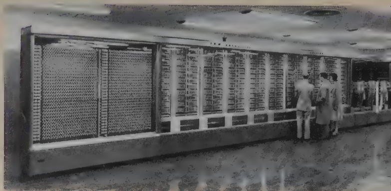
10 Howard H. Aiken, Ph.D. candidate at Harvard University, devises Mark I, the first large-scale automatic digital calculator
