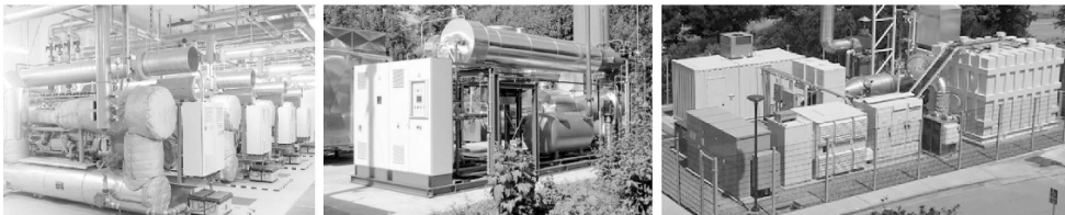
Figure 1.2 Combined heat and power plant; ORC plant; fuel cell power plant (from left to right)
