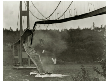
FIGURE 5.R.6 Collapse of the Tacoma Narrows Suspension Bridge
